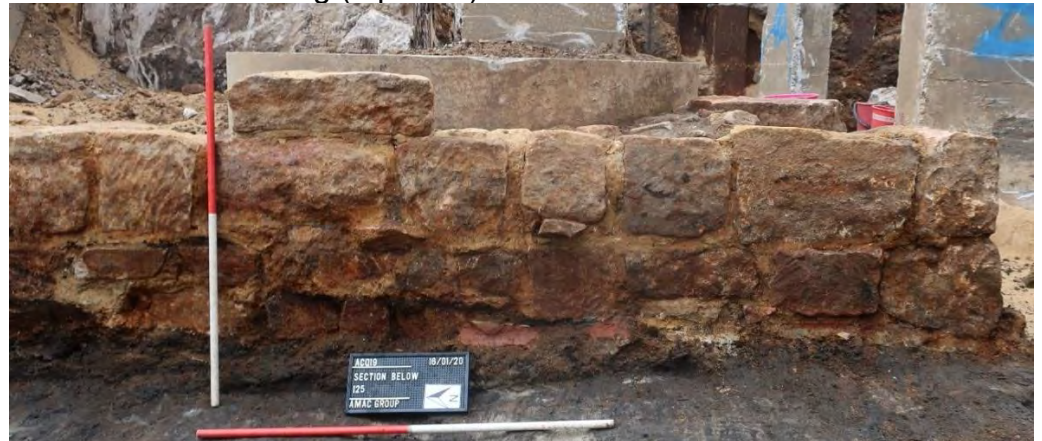
Sandstone wall footing (side view)
