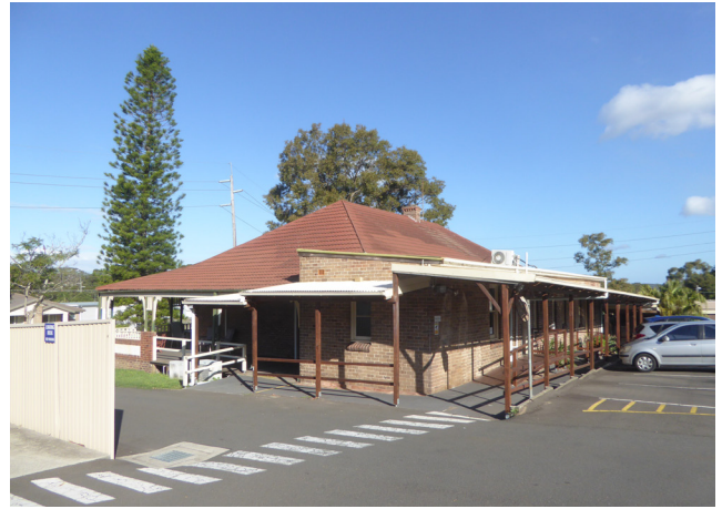
Figure 3.2 Skillion-roofed, single storey wing stretching across the back of the house, containing a number of services rooms and a covered walkway.
