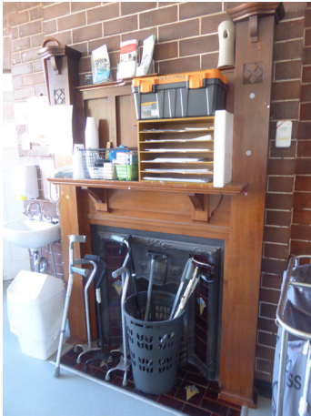
Figure 3.15 The existing chimney breast and fireplace (Item 9), located within the former gym area.
