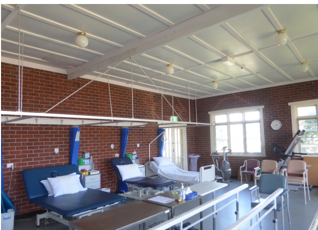
Figure 3.5 Internal view of the southern addition with facebrick internal walls and undecorated ceilings. The room is also referred to as a billiard room in the 1928 auction sale advertising.
