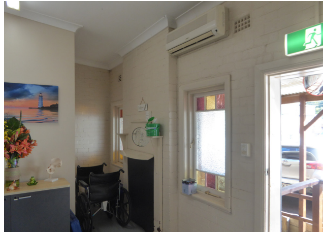
Figure 3.16 The relocated chimney breast and fireplace (Item 10), located within the rear later addition.
