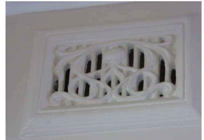
Figure 3.17 Existing decorative plaster air vents (Item 11), evident in the front portion of the building.
