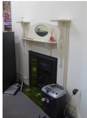
Figure 3.13 The existing chimney breast and fireplace (Item 7), located within the office.
