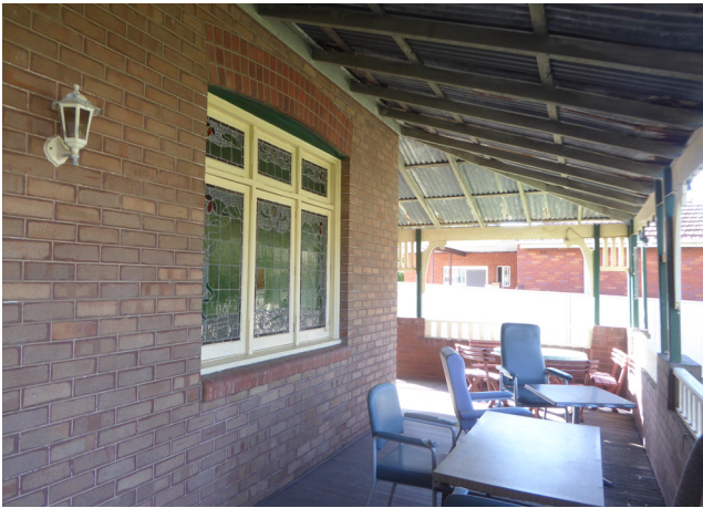
Figure 3.3 Polychromatic brickwork, and leadlight windows of the front verandah.
