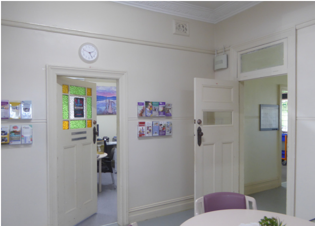
Figure 3.9 View to existing internal timber doors (Item 5).
