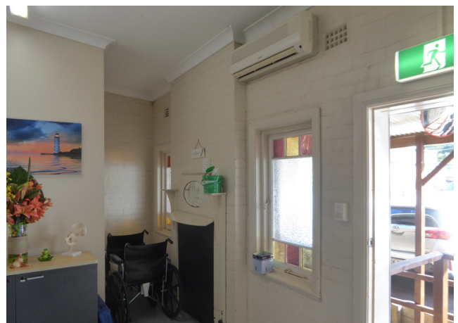
Figure 3.6 Room within the rear addition contains a decorative fire surround, relocated from elsewhere in the house.
