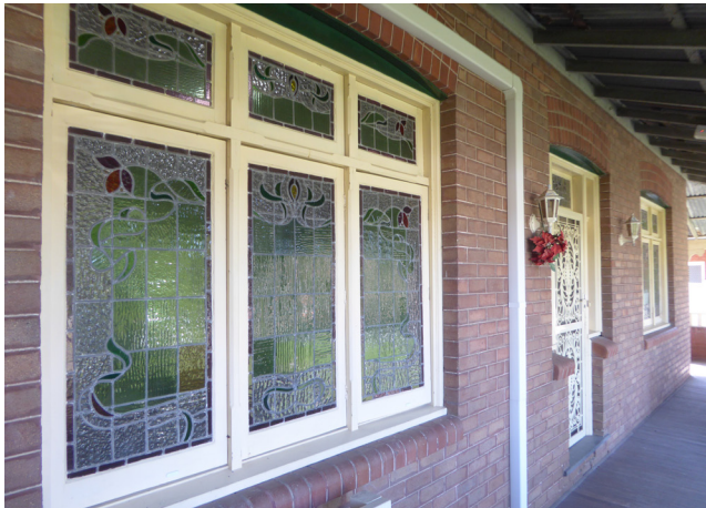
Figure 3.3 Close up view to the existing eastern elevation, including the stained glass windows (Item 2).
