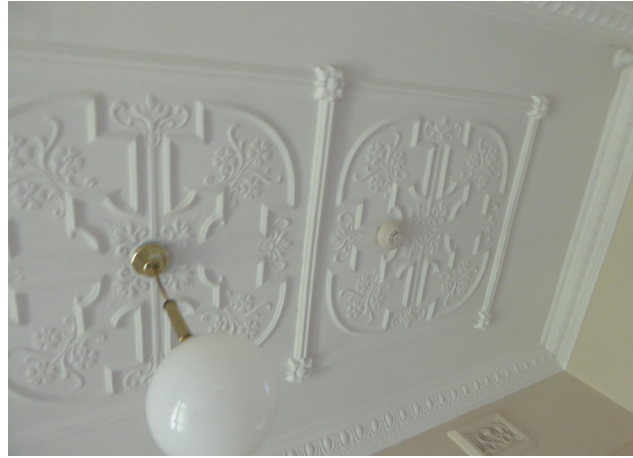
Figure 3.10 Existing decorative plaster ceiling within the entrance hall, note the pendant lighting (Item 6A).
