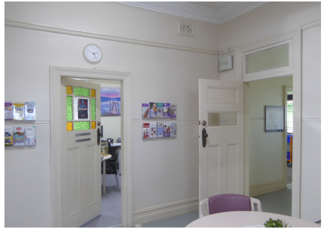
Figure 3.4 One of the internal rooms with access to the entry corridor from the front verandah.
