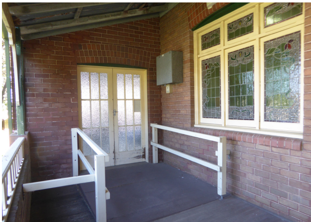
Figure 3.6 View to the timber framed swing doors providing access to the former gym, as accessed via the ramp.
