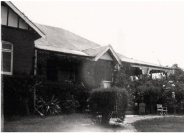
Image 12 Photograph of the dwelling, date unknown. Included in the Sutherland Shire Council Archives, MF003297. Source: Architectural Projects Pty Ltd., 65 Hotham Road, GyMEA: Heritage Assessment Review, March 2009, Figure 3.10.
